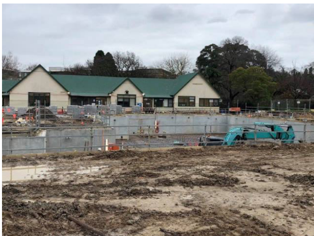
The groundworks for the new precinct
